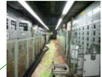
Unit1 Turbine Building Power panel
