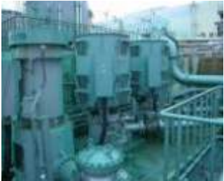
Unit1 PCV cooling sea water pump
