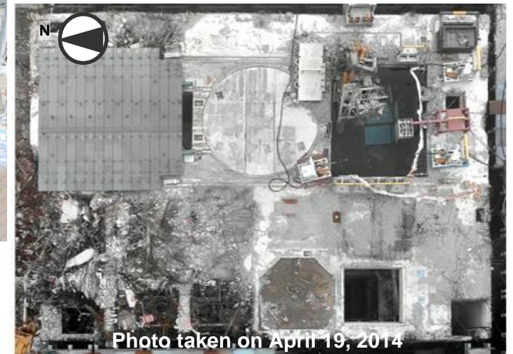
After removal of large debris
