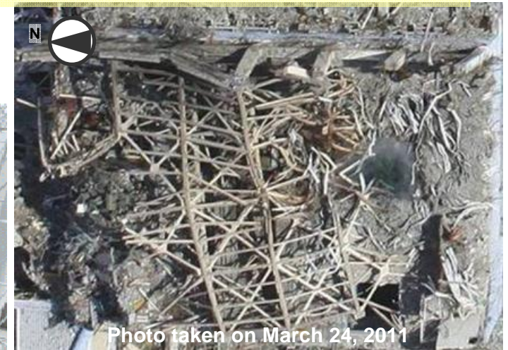
Before large debris removal
