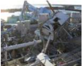
Unit5 Sea water pump area
