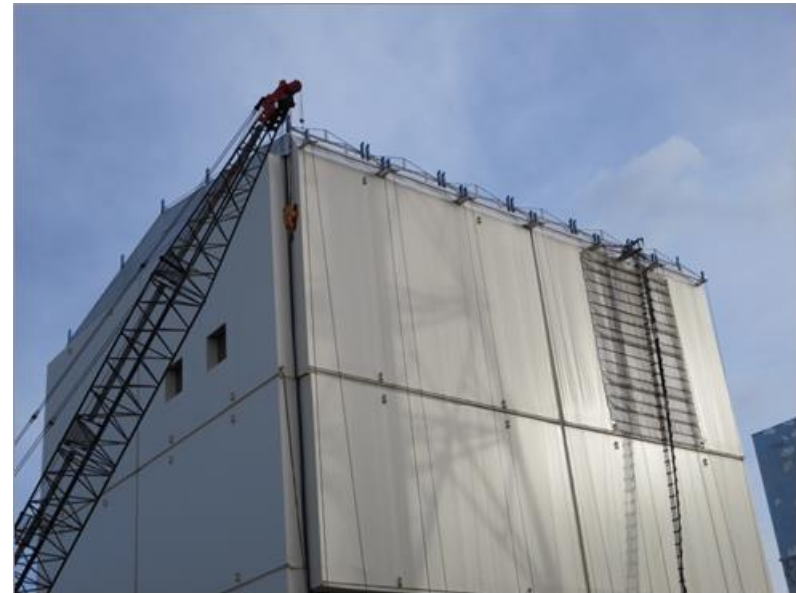
Completion of building cover structure Present
