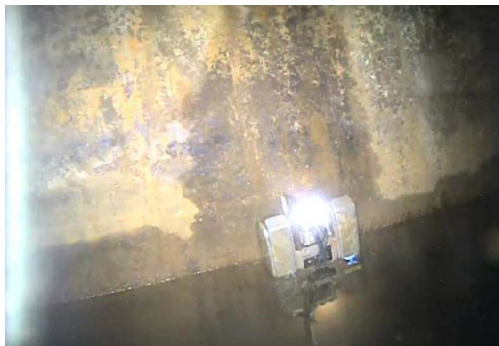
During the water level measuring
