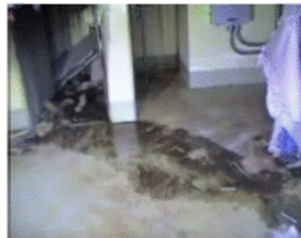
Water flow reduction confirmed (on Jan. 21)
